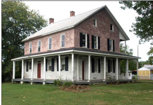
Justice William Smith's house before 2011 dismantlement (lower limestone story was original house)
